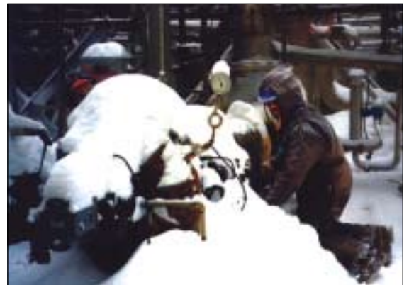
Right: Onsite service of a pump in difficult conditions
