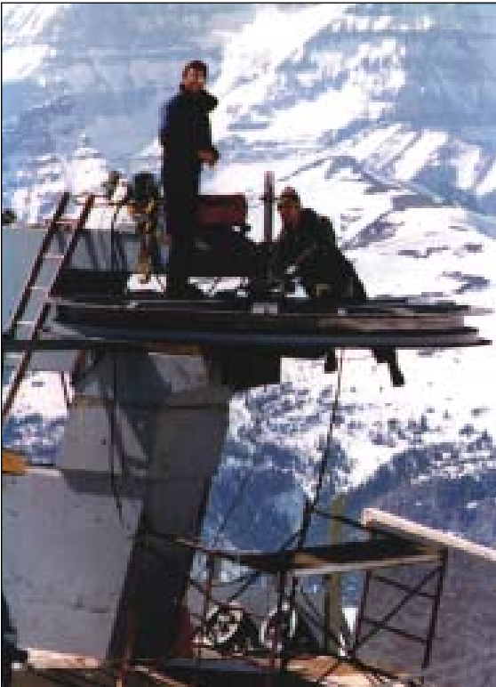
Top: Wash drum seal resurfacing
