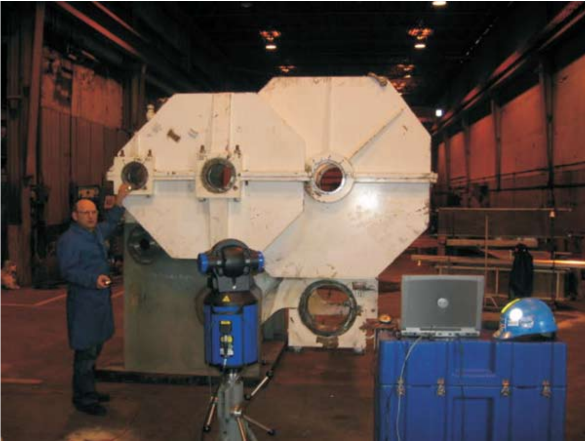
Gearbox bore alignment - During overhaul, boring tools are aligned prior to boring to ensure that bores are set precisely parallel with each other and to the correct spacing.
